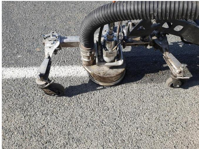
**Blasting.** Abrasive blasting can be carried out using various blasting medium including steel, garnet and glass. The system should incorporate a recycle process where the blasting medium is recycled into the equipment and used continuously through the blasting process
